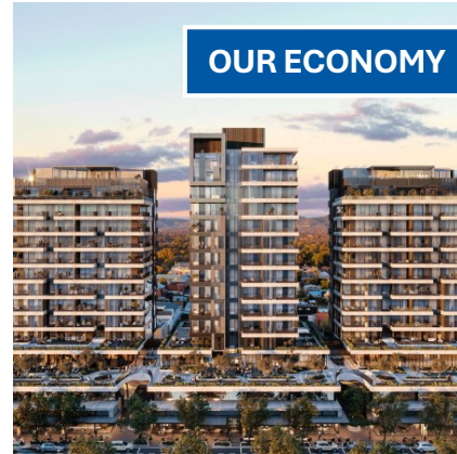
88 O'Connell Project Delivery
